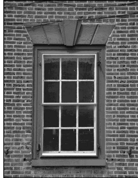
Figure 56: Historic window at the Mitchell House. The same type of wooden lintel can be found on several buildings in Elkton.
