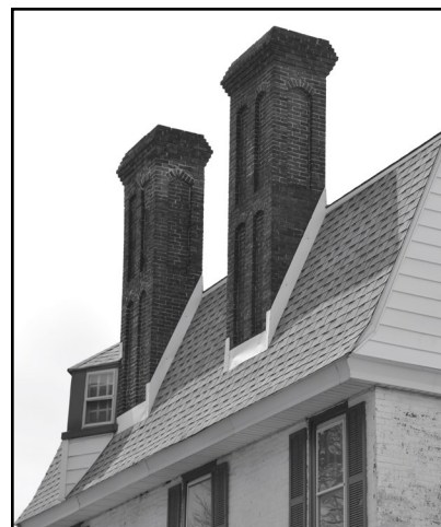
Figure 67: Chimneys with decorative corbelling should be retained.
