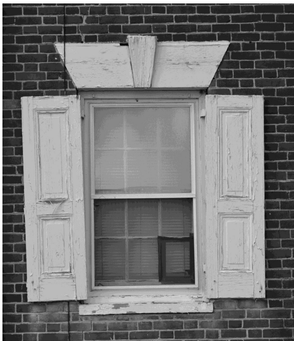
Figure 48: Example of peeling, delaminated paint. Shutters such as these should be detached and failed layers of paint removed before being repainted. These oversized wooden lintels are a distinctive Elkton feature.
