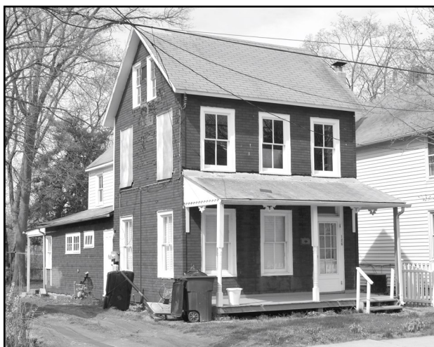
Figure 44: Asphalt siding to imitate brick was installed on this historic house, c. 1930. This nineteenth-century house likely originally had wood clapboard siding.
