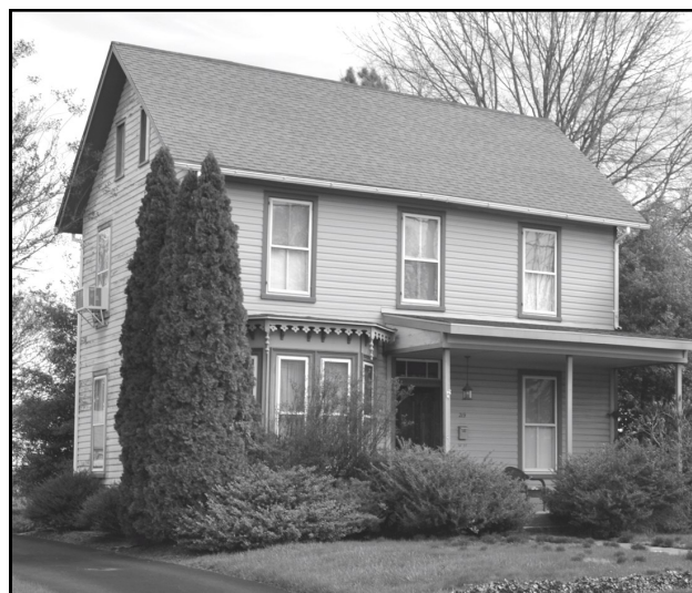
Figure 47: The scale and profile of the vinyl siding used on the front of this historic building matches the original wood clapboard siding visible on the side of the house in scale and profile. The building's original wood trim was left exposed.
