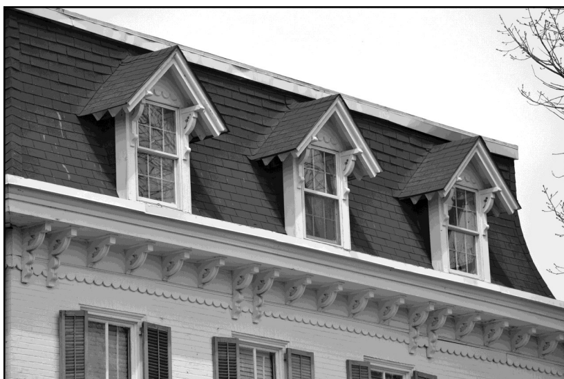
Figure 66: Dormers are an important feature of roof systems that need special attention and regular maintenance.
