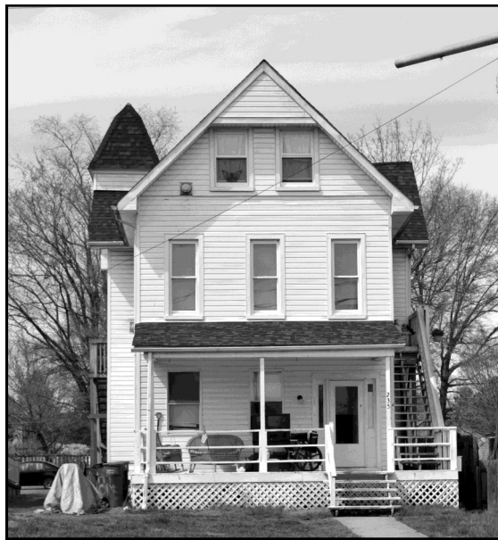
Figure 46: Vinyl siding obscures much of this late nineteenth-century building's detailing, such as window frames, corner boards, and vergeboard.
