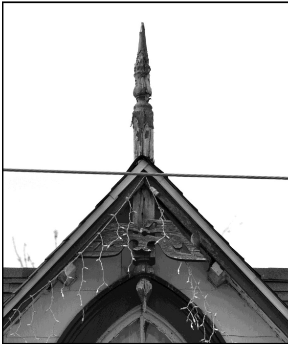
Figure 50: Wood details should be painted regularly to keep them in good repair.
